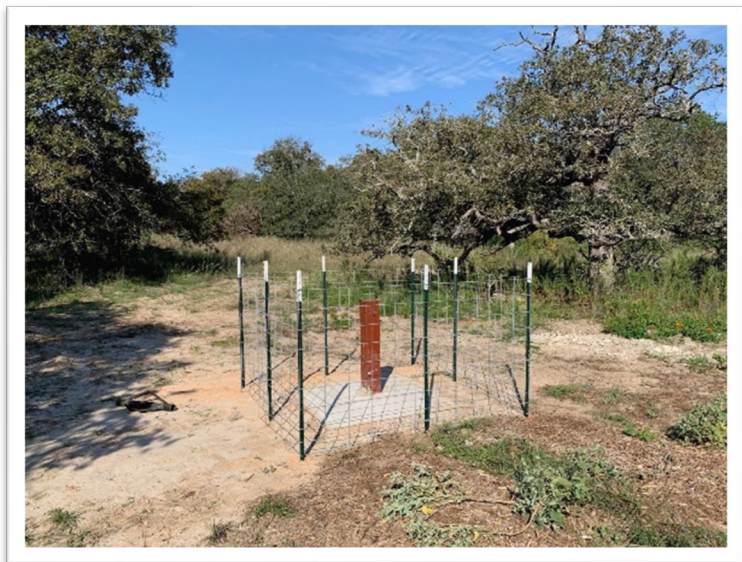
Fence constructed around wellhead at MWCZ-1B
